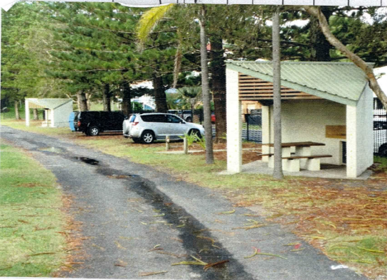
6. Masonry bbq shelters (3)
